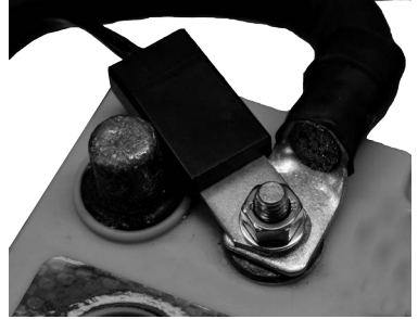
Fig 2.5(b) Temperature Sensor Installation
